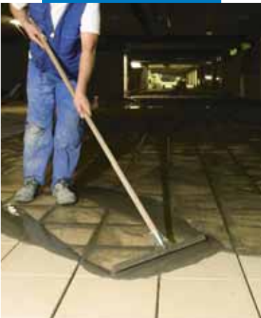
Application of Maxifuga using a rake
