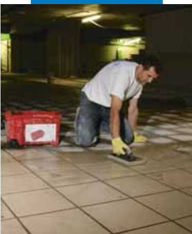
Cleaning surface with Scotch Brite® pad
